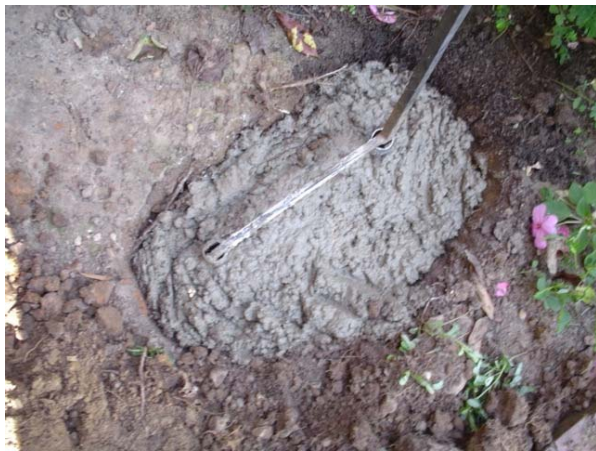
Pipe/concrete stability solution.
