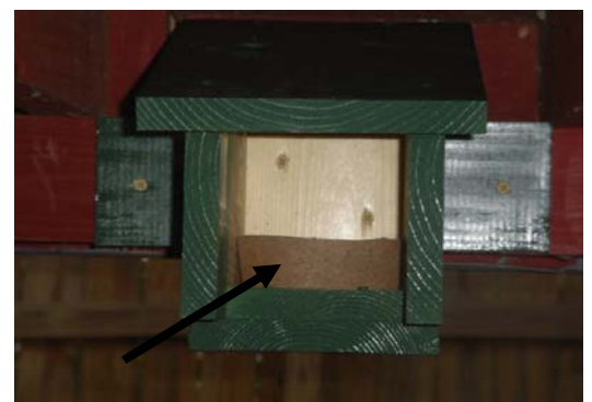
Latest generation nesting ledge for smaller birds. The rear-pivot floor swings downward for easy cleaning. This is necessary due to the lip on the front of the floor. Notice the use of the molded wood-fiber nesting cup.
